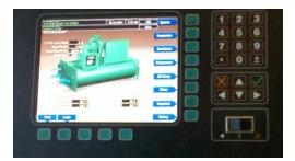
Figure 3: Chiller control panel
