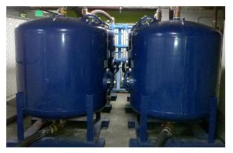
Figure 6: Carbon filters used to treat groundwater
