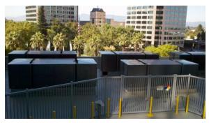
Figure 16: Fuel cells on roof at Adobe Systems
