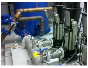
Figure 4: Domestic water pressure station
