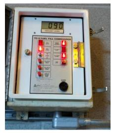
Figure 1: Enclosure with generator fuel indicators
