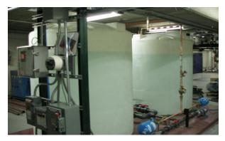
Figure 9: Cage pre-wash water storage tanks
