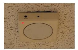
Figure 6: Motion sensor to turn lights on/off
