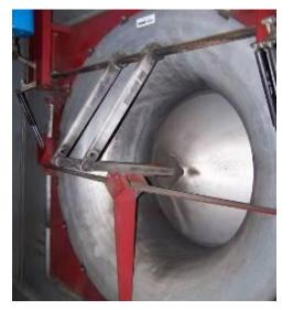
Figure 12: Econo-cone within the 68,000 CFM air handler
