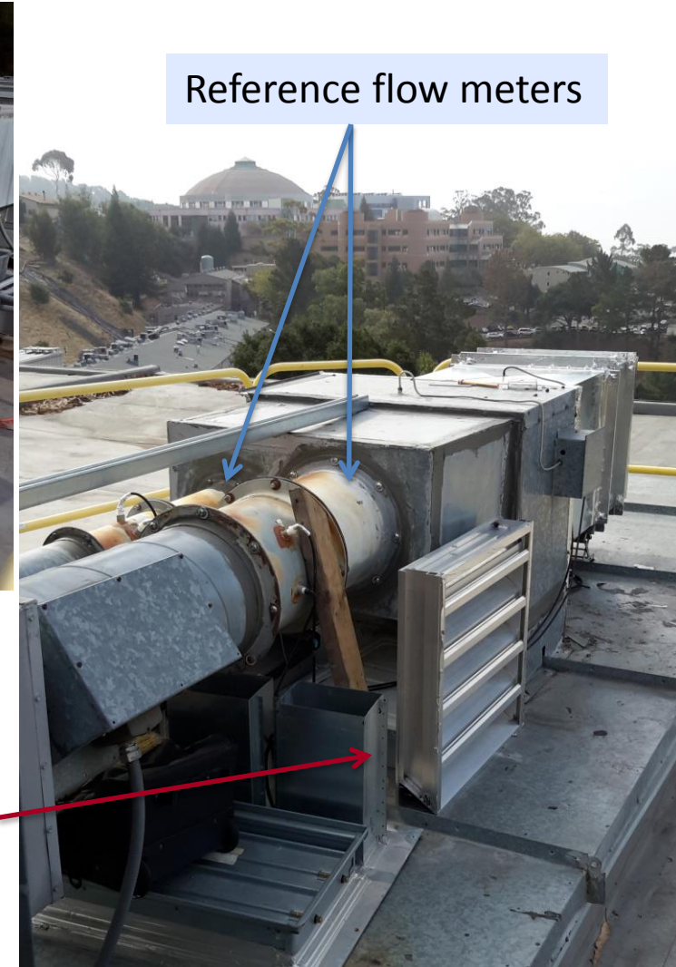
Typical low velocity horizontal-blade louver that directs air upwards
