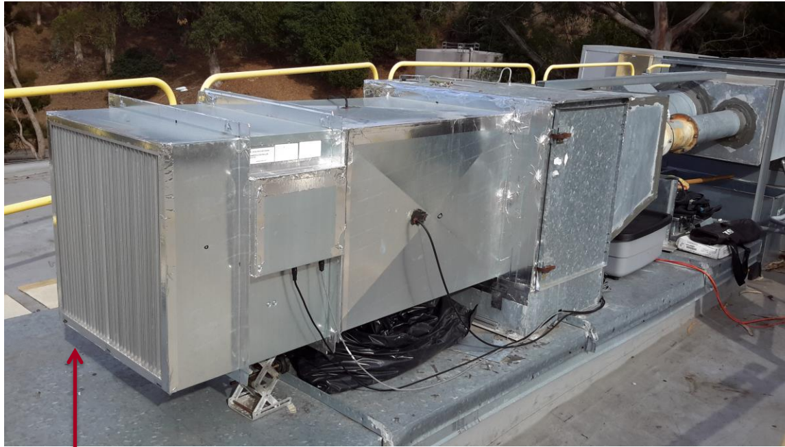
Higher velocity vertical-blade louver that directs air to one side
